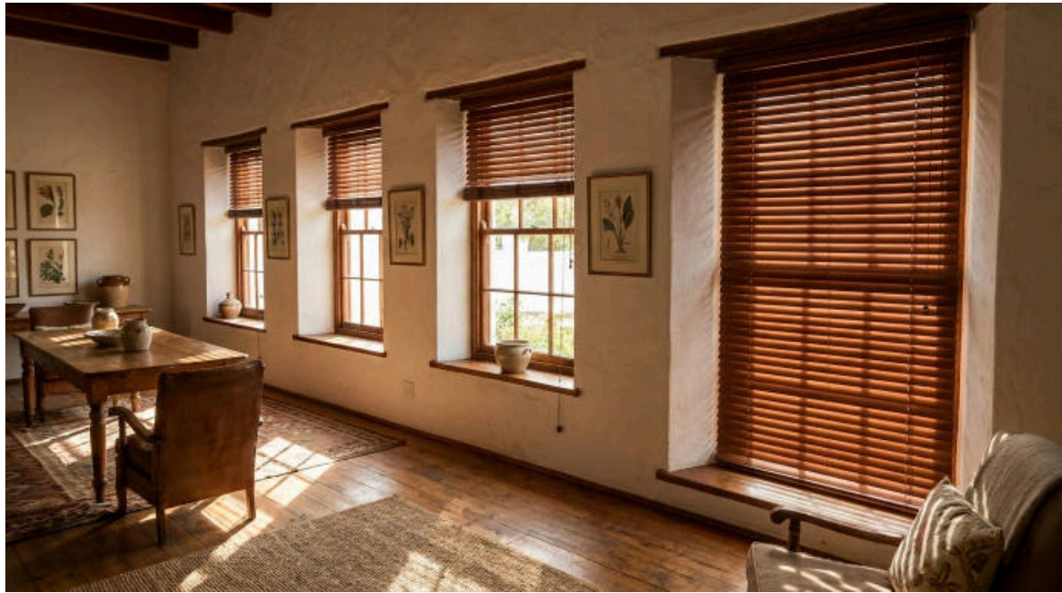
Four openings in one wall, four different tilt angles. Deep reveals let each window be tuned separately without anything showing on the facade.
