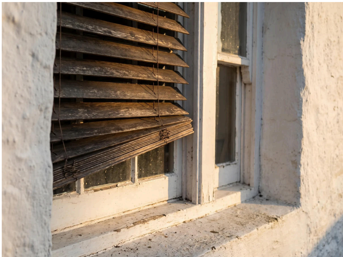
Where the blind meets the joinery is where a heritage job is won or lost — the fixing goes into the plaster and masonry, not through two-hundred-year-old timber.
